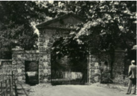
Entrance archway in 1950, prior to collapse.
